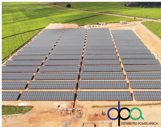
Tanganda tea company solar plant by (DPA) Distributed Power Africa
